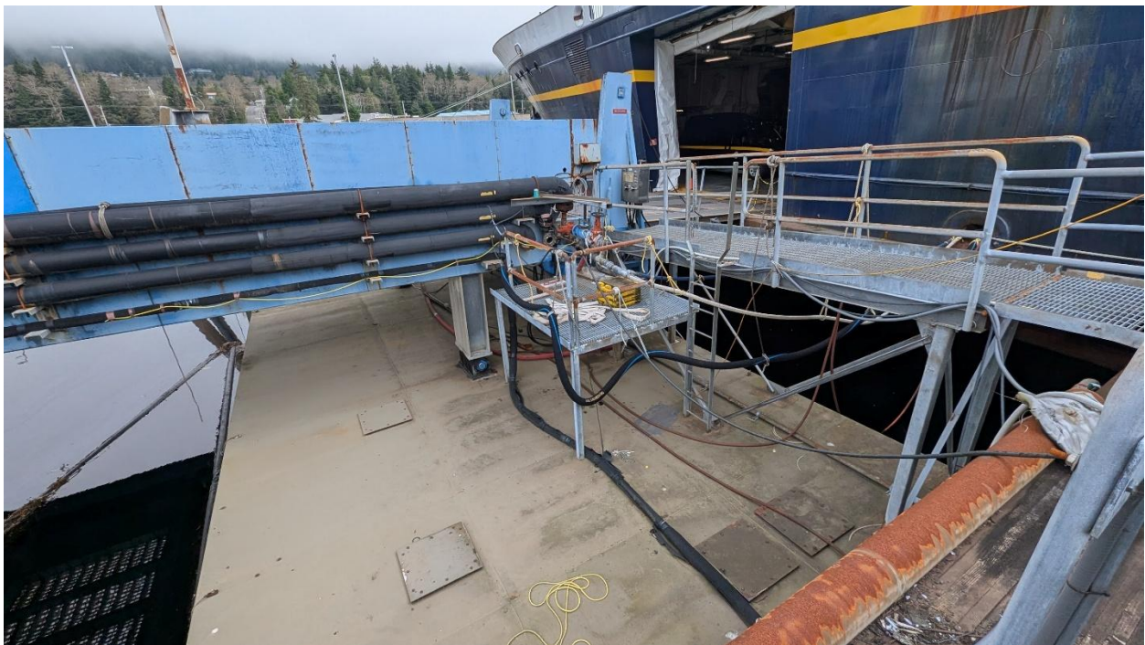
Figure 6- Berth 2 Ramp, Float and Apron, Observed October 2025
