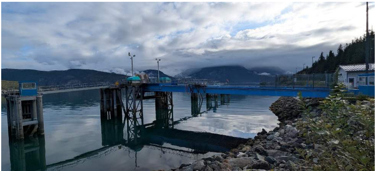
Figure 16- Haines Terminal Ramp and Lifts, Observed October 2025
