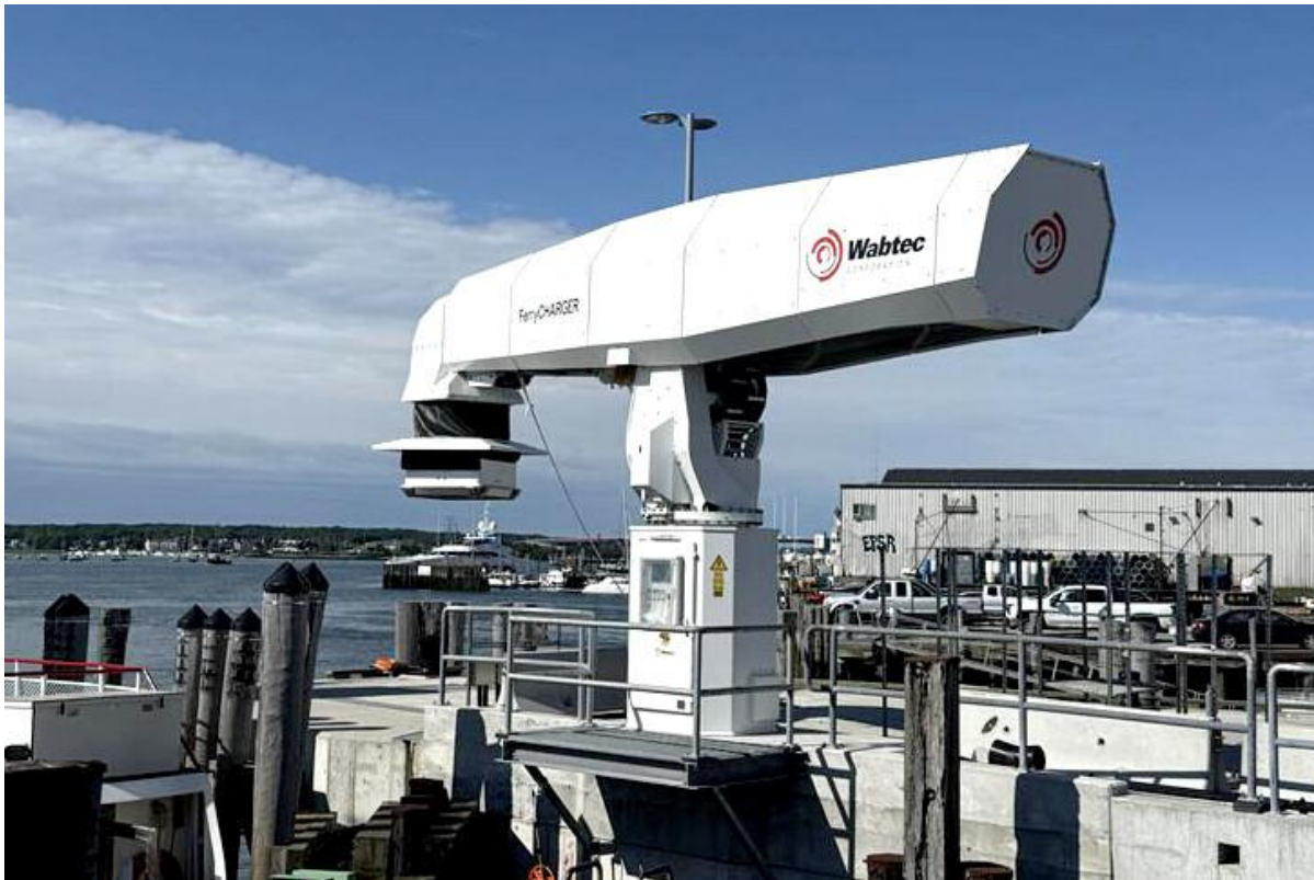
Figure 4- Charging Arm for Casco Bay Ferry, larger than the systems anticipated to support the HE Ferry 3
