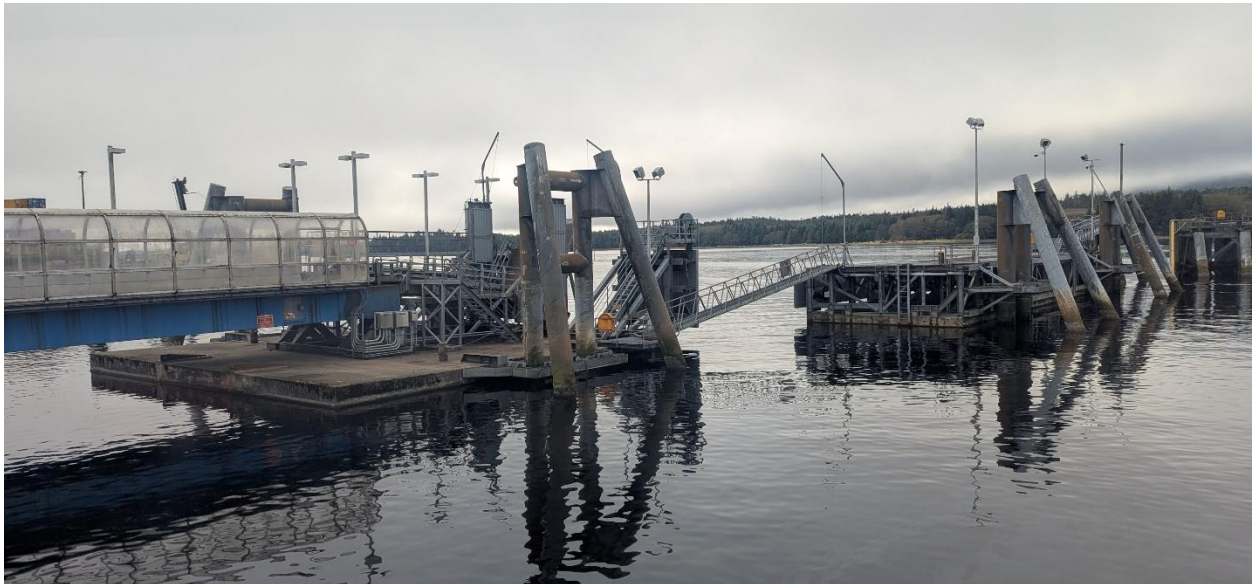
Figure 9- Berth 3 Float, Ramp and Fendering Float, Observed October 2025
