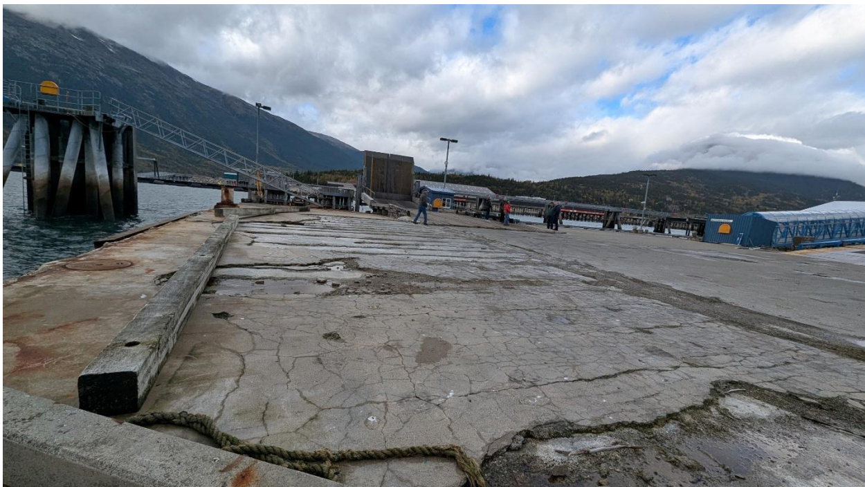
Figure 18- Skagway Concrete Float & Apron in Background, Observed October 2025
