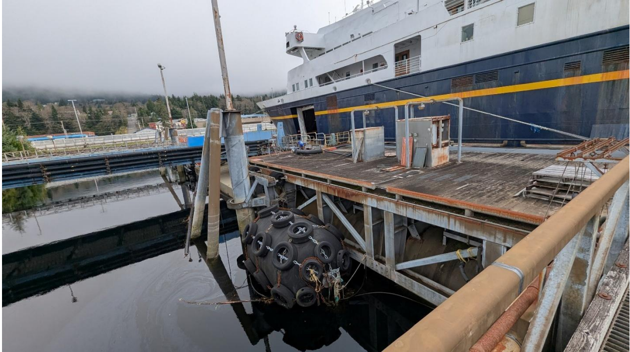
Figure 5- Berth 2 Fender Float & Ramp, Observed October 2025
