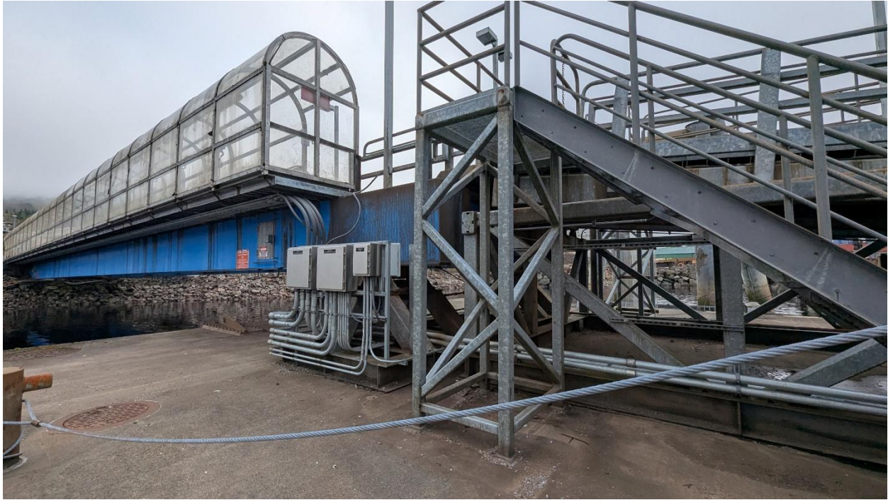
Figure 8- Berth 3 Float and Ramp, Observed October 2025
