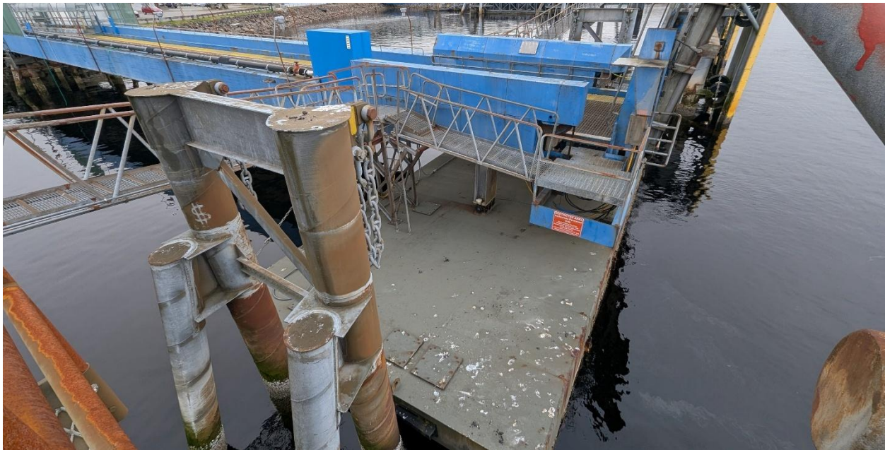
Figure 3- Berth 1 Float, Ram and Apron, Observed October 2025
