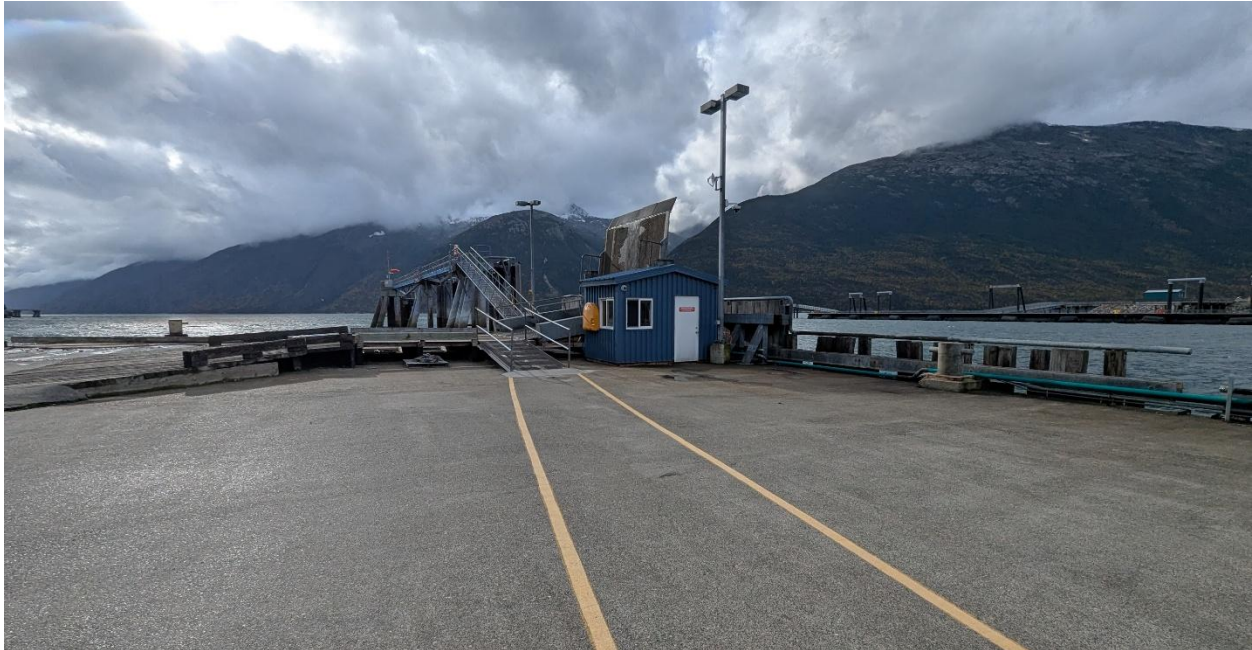
Figure 19- Apron on the Skagway Float, Observed October 2025
