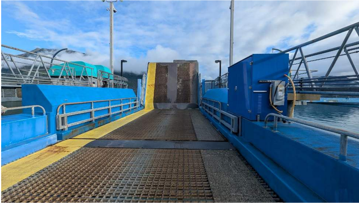
Figure 17- Haines Marine Terminal Loading Ramp, Observed October 2025
