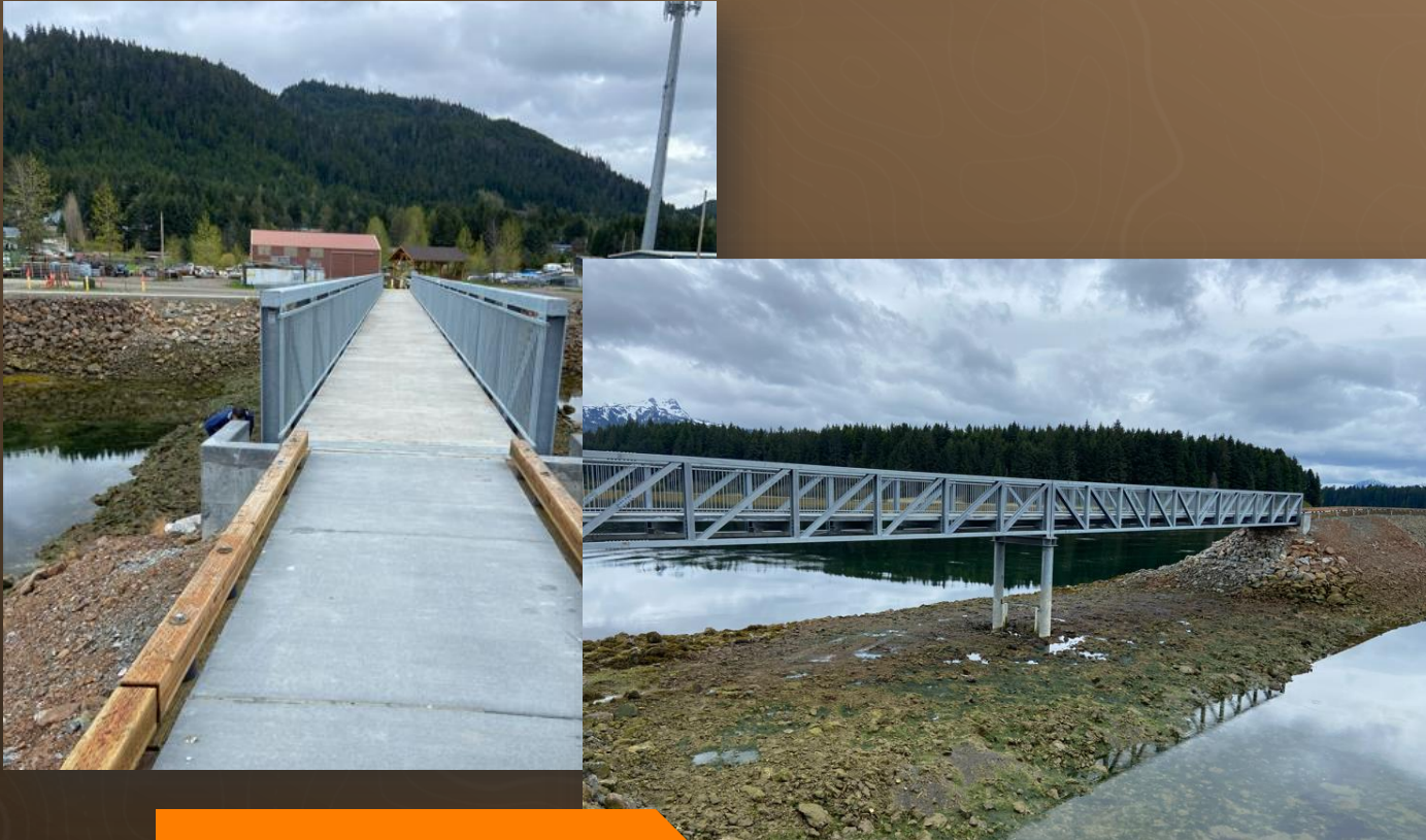
New pedestrian bridge structure to shore
