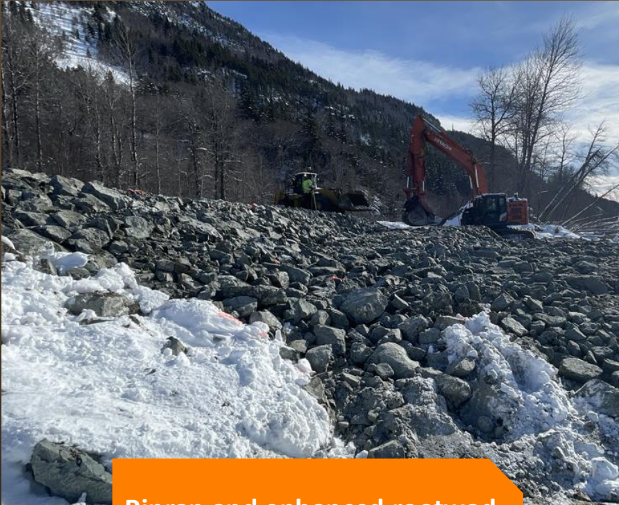
Riprap and enhanced rootwad embankment installation
